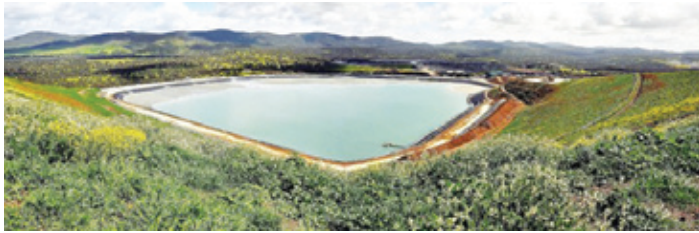
Fig. 1: Field photograph of Aguablanca nickel and copper mine tailings storage facility in a valley depression in Spain [Photo source: Wikipedia]
