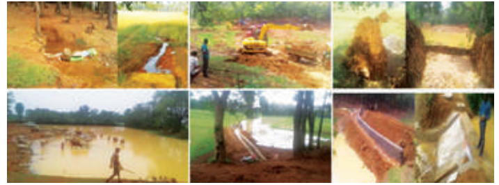
Fig 9: Process for developing Spring Based Water Harvesting Structure for Agriculture
