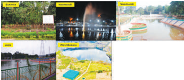
Fig 8: Rainwater harvesting structures across Tata Steel's mining locations
