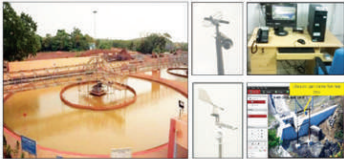
Fig 7: Effluent Treatment Plant (ETP) and Water Monitoring at Sukinda Chromite mine
