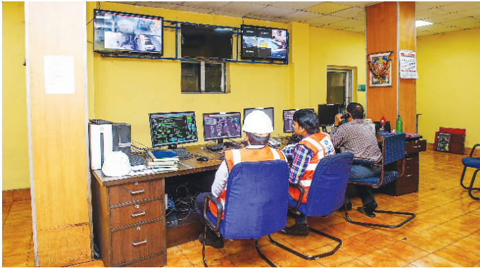
Centralised Control Room
