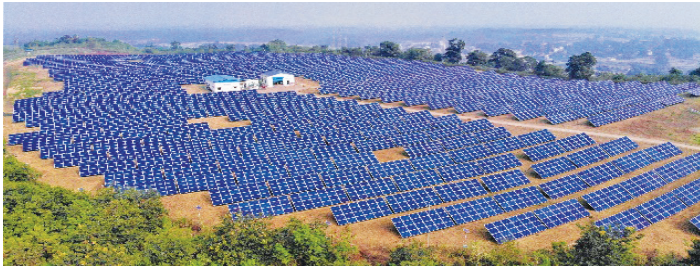
Solar Power Plant at Noamundi
