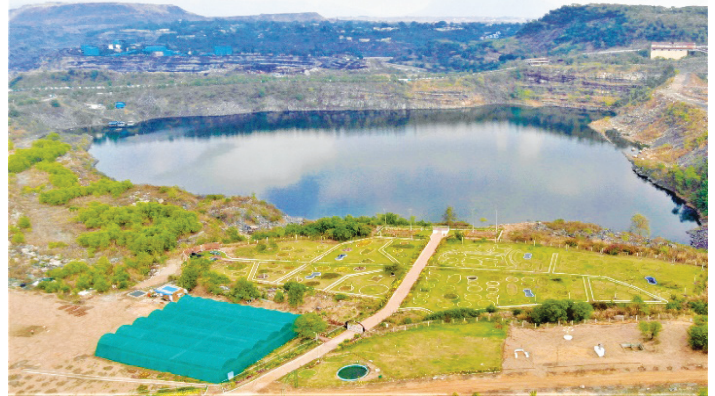
Water Reservoir for Rainwater Conservation
