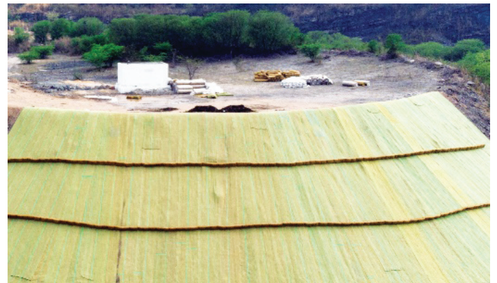
Geo Coir Matting - Before
