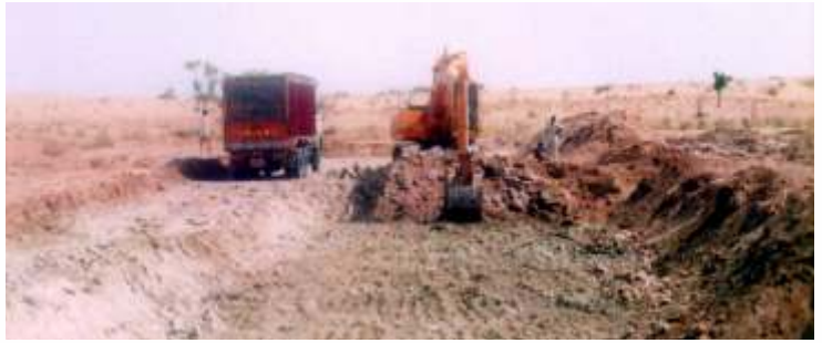
Removal of Gypsum
