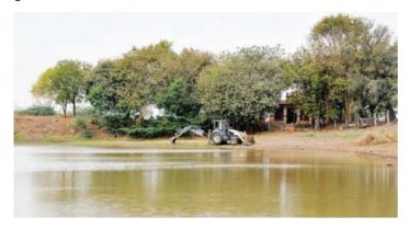
Check dams can strengthen the groundwater recharge, control the water velocity, and reduce the soil erosion of the surrounding area. To increase water conservation of the surrounding area, GMDC regularly undertakes Check dam deepening work.
