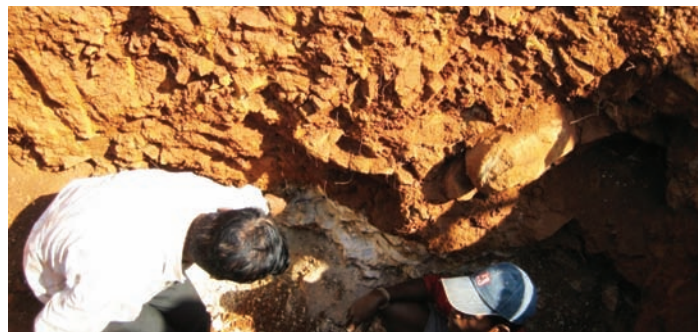
Fig. 1. Open trench mining of mineralised pegmatite (white body), intruding a meta-basic rock (brown-coloured). The depth of the trench is about 3.5 metres vertically below the surface. Note black crystals of columbite-tantalite and green mica in trench floor. Location. Bastar pegmatite belt, Chhattisgarh.
