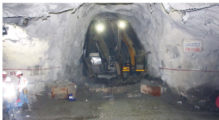
Figure 4. Monitoring of ground vibration generated due to working of rock-breakers
